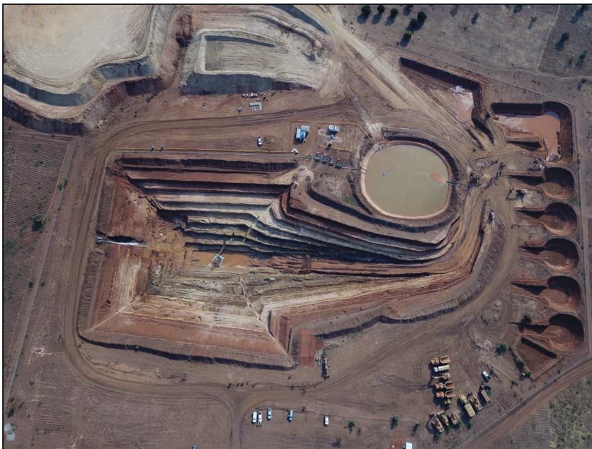
Figure 7: Overview of the hydraulic mining trial
