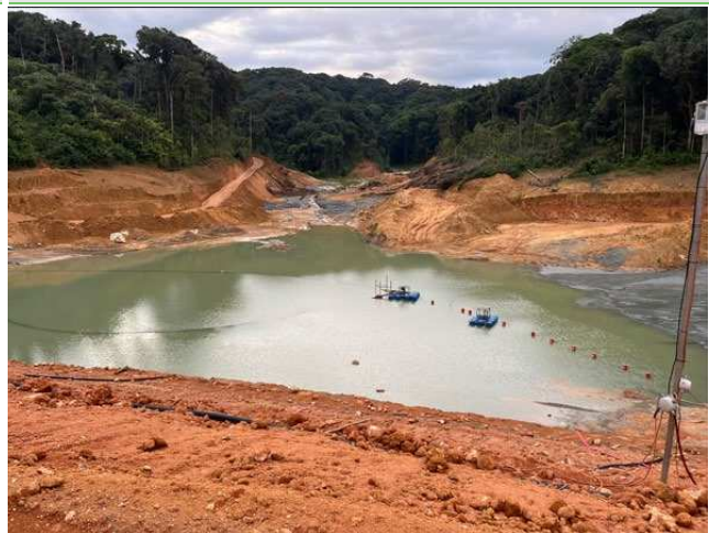
Exhibit 7: To Omega – the No. 2 Tailings dam ready for deposition
